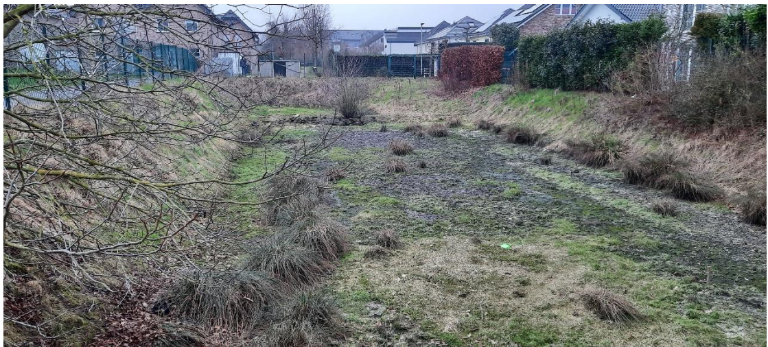
Figure 13 Small detention basin for buffering rainfall water in Herzogenrath-Bierstraß (photo: B. Becker)
